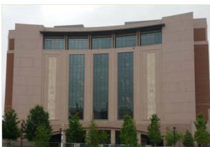
Tom Vandergriff Civil Courts Building 100 N Calhoun Street
