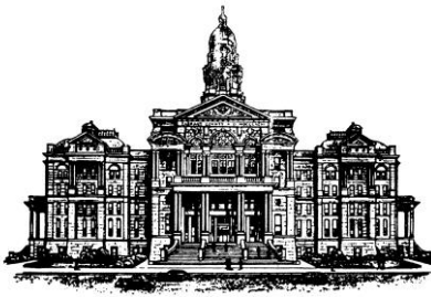
Tarrant County 1895 Courthouse
