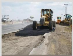
Pavement repair on Bonds Ranch Road in preparation for new asphalt surfacing.
