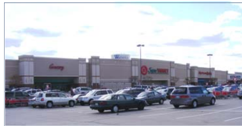
Watauga Towne Crossing
