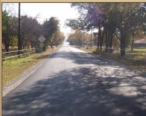
Completed project - asphalt overlay on a section of Randol Mill Road
