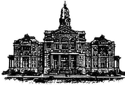
Tarrant County 1895 Courthouse
