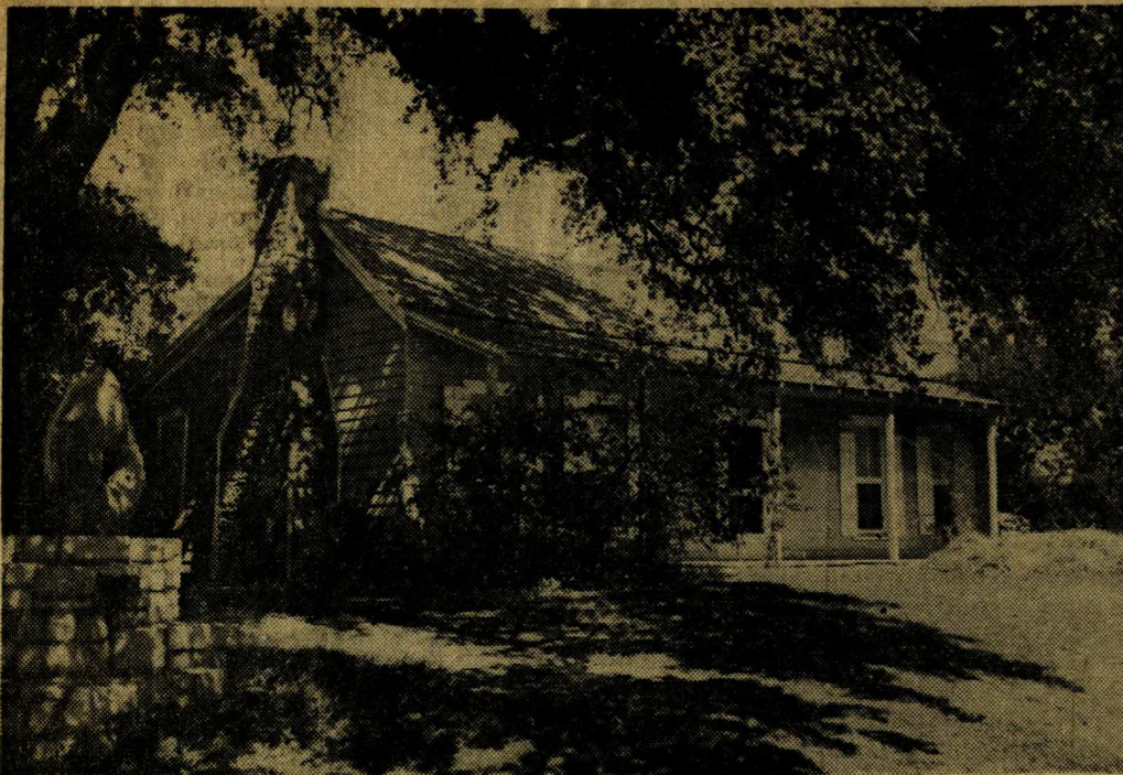
READY FOR VISITORS —Van Zandt Cottage in Trinity Park, a landmark in the development of Fort Worth, has been re-
