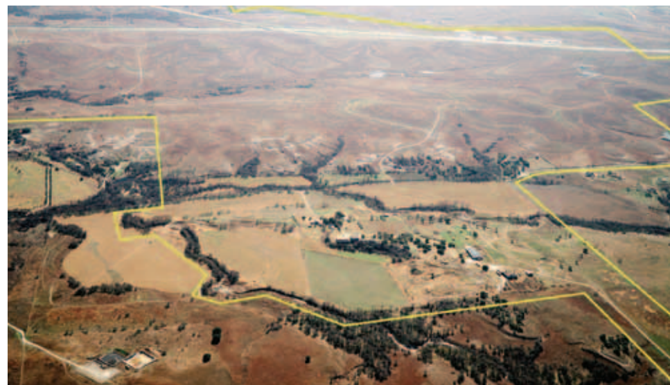
Aerial photograph looking south toward I-20
