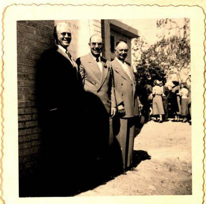
Buford Johnson, T. E. Durham and John Linguist laying cornerstone 1949
