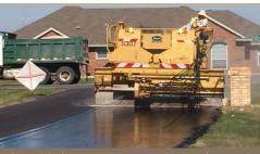
Pictured above: Improvements made to Haslet Heights and Country Ridge Estates using the chip seal process. During this process, liquid asphalt is applied to the surface and is followed by a layer of crushed gravel which is embedded by the pneumatic roller. After a few days, the excess rock is swept up.
