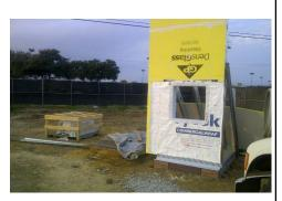
Mockup - Left to right you can see the crated stone, the concrete finishes which will soon have some terrazzo added and the studs and wall opening where a window will be installed.
