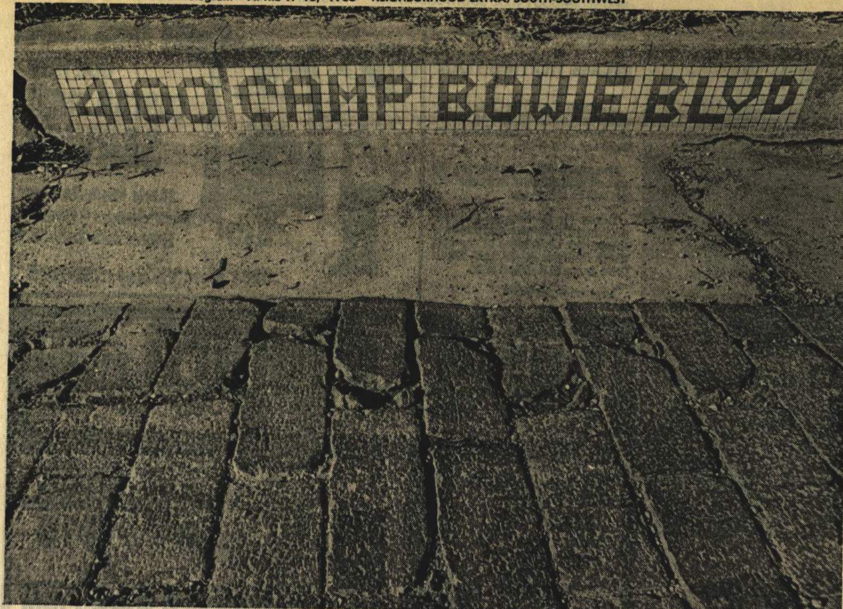
There's a shortage of brick to replace the old, worn and broken bricks on Camp Bowie Boulevard. Star-Telegram
