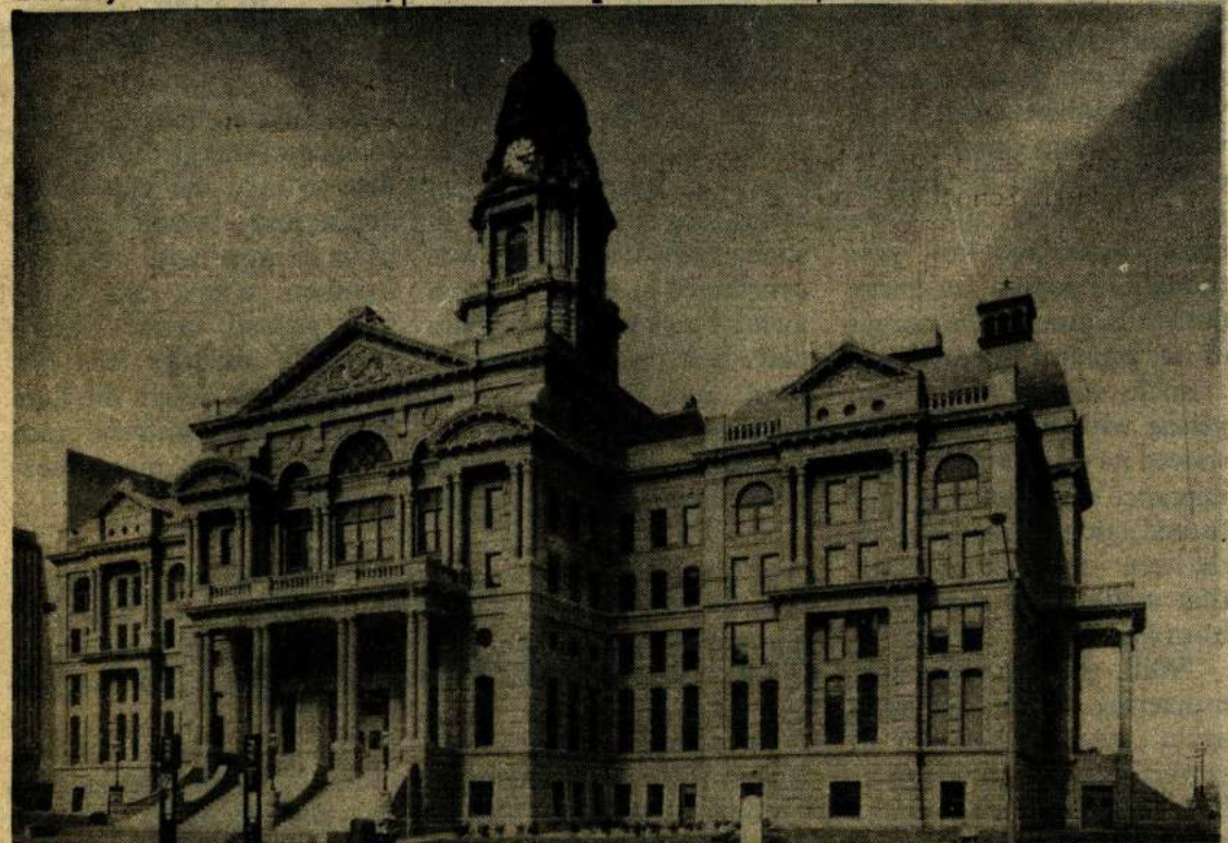
THE TARRANT HOUSE OF COURTS - Tarrant County's majestic courthouse is constructed of gray granite from the granite mountains of Burnett County. It is trimmed with Texas marble from the same county and features a copper roof. The design favors both French and Italian Renaissance architecture. The structure rises 193 feet at its highest point and covers 114,211 square feet of floor space. Photo by Bob Guarnieri
