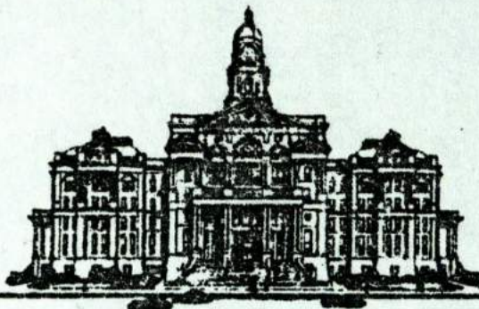
TARRANT COUNTY COURT HOUSE FORT WORTH, TEXAS
