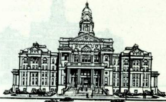
TARRANT COUNTY COURT HOUSE FORT WORTH, TEXAS
