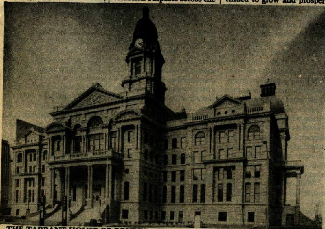
THE TARRANT HOUSE OF COURTS - Tarrant County's majestic courthouse is constructed of gray granite from the granite mountains of Burnett County. It is trimmed with Texas marble from the same county and features a copper roof. The design favors both French and Italian Renaissance architecture. The structure rises 193 feet at its highest point and covers 114,211 square feet of floor space.
