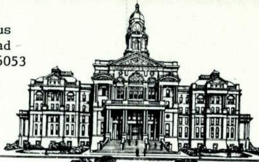
TARRANT COUNTY COURT HOUSE FORT WORTH, TEXAS
