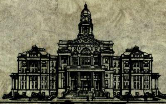
TARRANT COUNTY COURT HOUSE FORT WORTH, TEXAS
