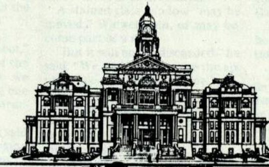
TARRANT COUNTY COURT HOUSE FORT WORTH, TEXAS
