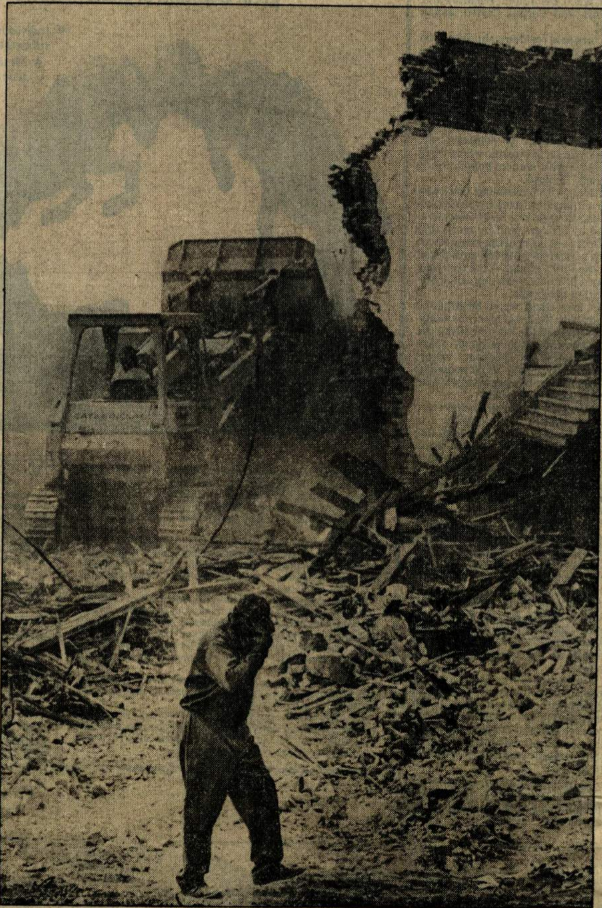
WALLS COME DOWN ... George Williams shields his eyes during demolition
