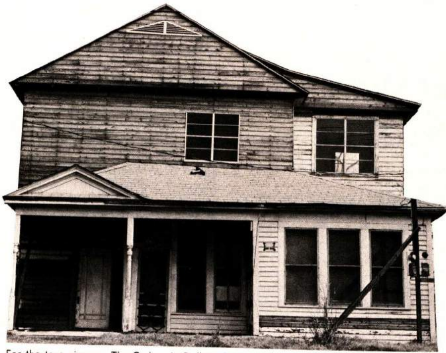
For the true pioneer, The Cedars in Dallas offers opportunities for extensive restoration.
