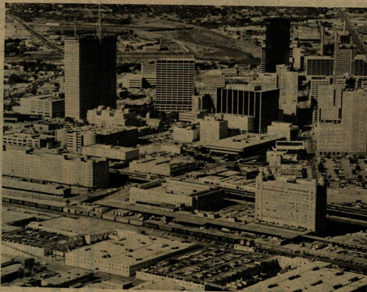
MORE DOWNTOWN CHANGES —The Fort Worth skyline isn't the only thing to change downtown when the new central business district
