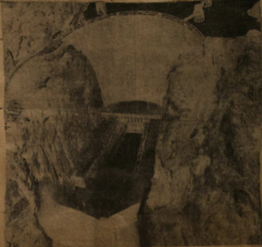
BOULDER DAM ENGINEERS CREATED ONE OF THE LARGEST MAN- made waterfalls ever seen when they released more than 30,000,000 gal- lons of water from Lake Mead through the dam's giant outlet valves 183 feet above the bed of the Colorado River in an inspection test.
