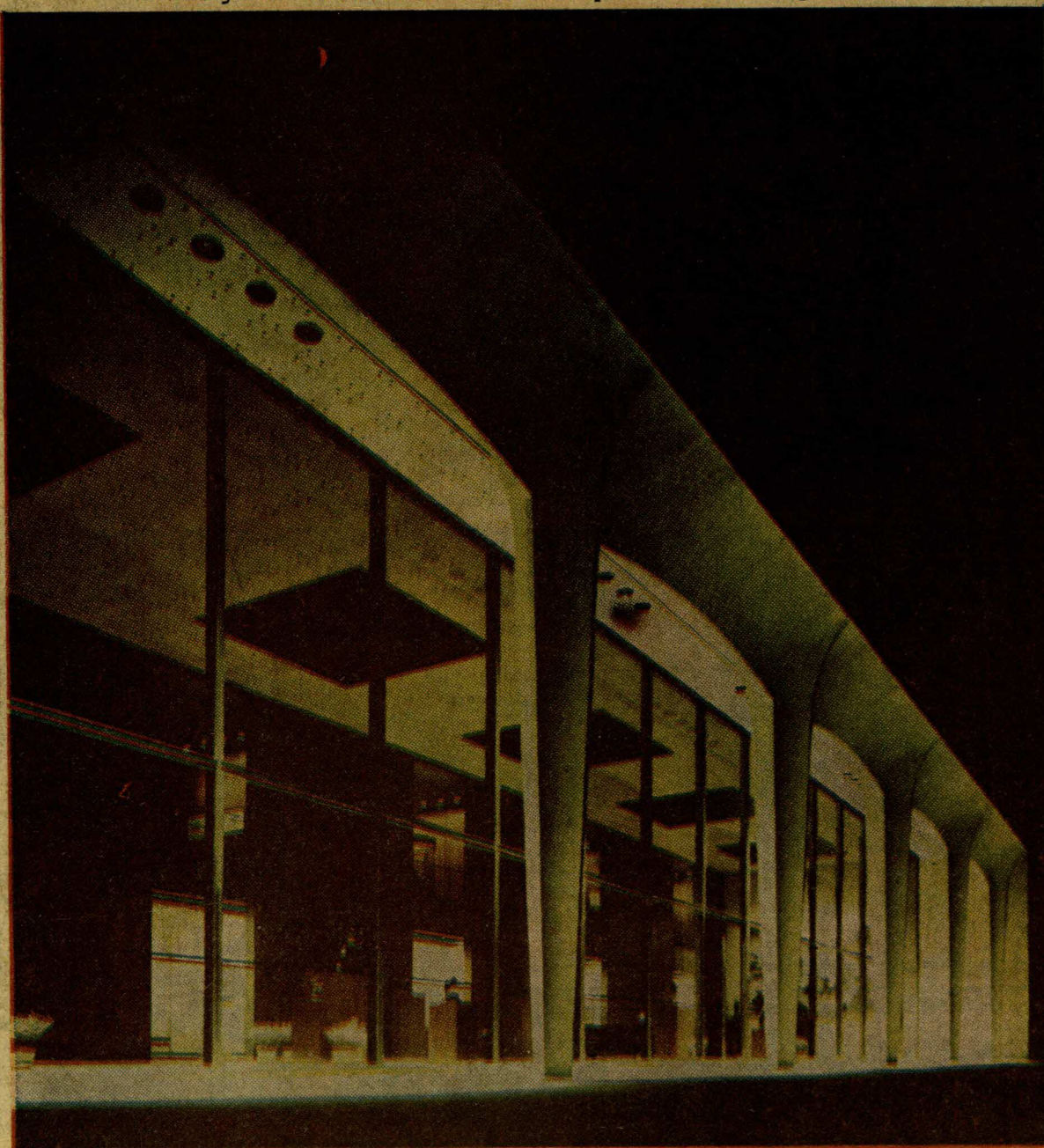
Like the oldtime Indian lodges, the Amon Carter Museum of Western Art faces the rising sun. The structure is described by its architect, Philip Johnson.
