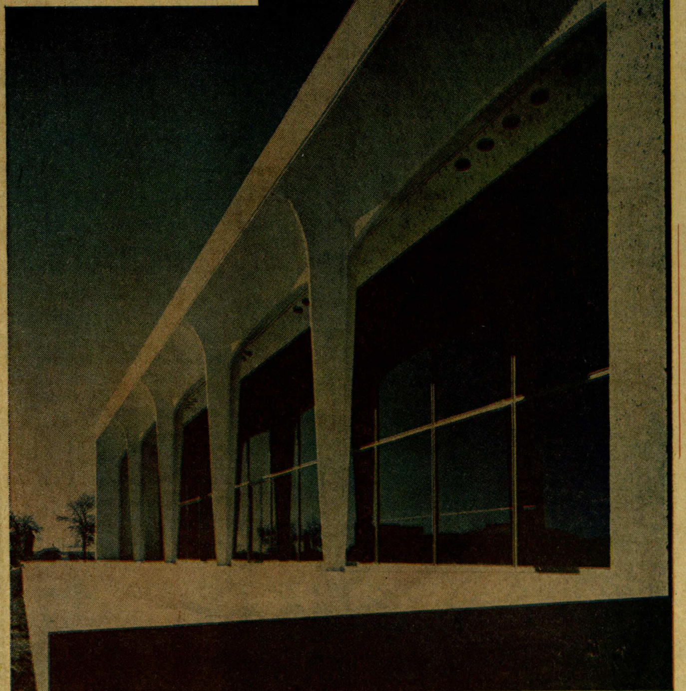
"The five segmental arches on tapered columns form an open porch overlooking terrace areas, a shaded place looking on sunny openness."
